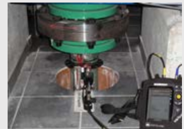
Fig. 4: Mobile load measurement on a small hydroelectric asset
