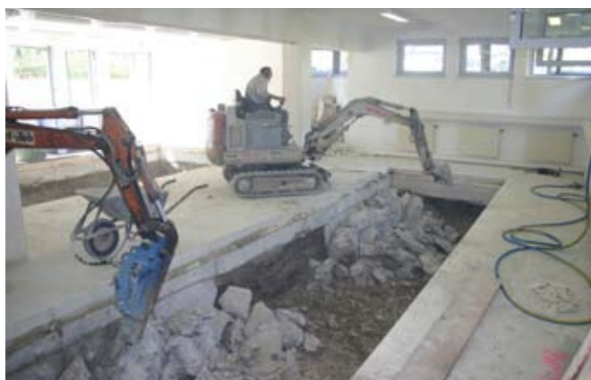
Despite the heavy excavation works, normal production operation continued unabated
