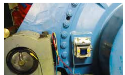
Image 6a (top) and 6b (bottom): Mounting of the laser/receiver unit, on the left on the main bearing, on the right on the gear for determining alignment targets
