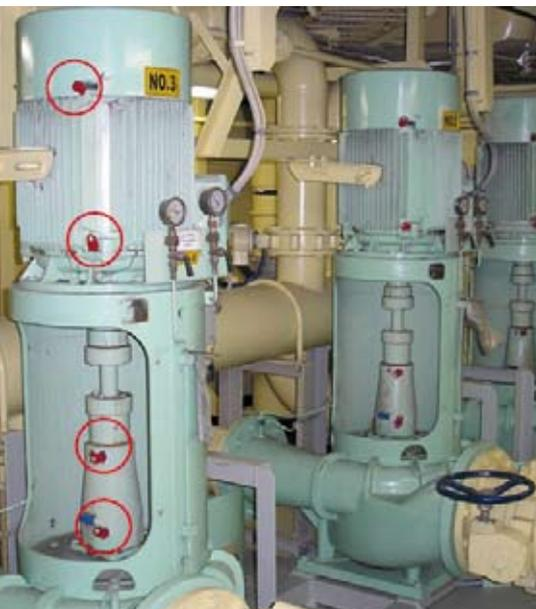
Vertical pumps equipped with 4 VIBCODE® measurement locations each
