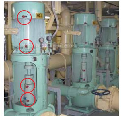
Fig.4: Vertical pumps equipped with 4 VIBCODE® measurement locations each
