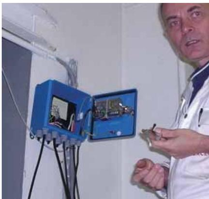
Fig.3: The VIBNODE® online condition monitoring system was installed temporarily
